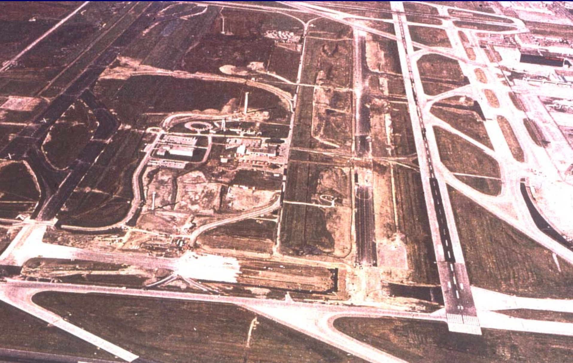
GTA 1998 NEW TAXIWAY AND RUNWAY ASPHALT PAVEMENTS UNDER CONSTRUCTION
