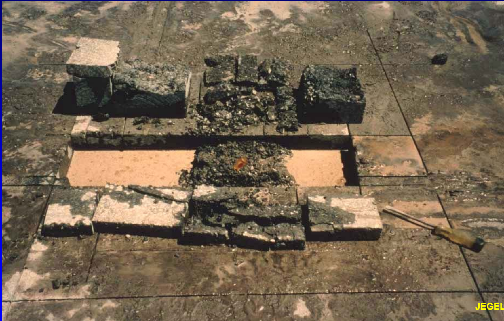
UREA DAMAGE TO HMA WITH A MOISTURE SUSCEPTIBILITY PROBLEM, DND GREENWOOD
